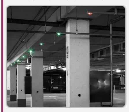
The Parking Guidance System allows free spaces to be quickly and easily located by using sensors connected to a LED coded systems, which shows a green light for available parking spaces, a blue light for handicap available spaces, and a red lights for occupied spaces.
